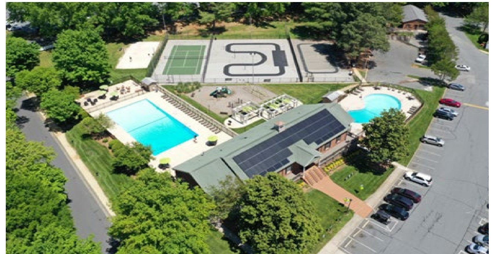
Solar panels reduce costs for common area electricity. Shown at Gardens at Country Club in Winston-Salem, NC
